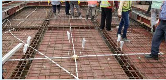
**Reinforced slab structure with embedded strain gauges before concreting**
