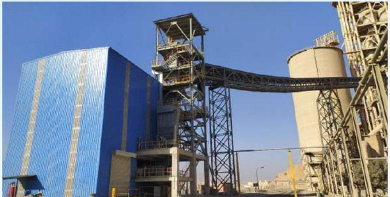
Commissioned system at site for storing, handling, and feeding tyre chips into the calciner
