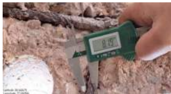
Measurement of existing rebar diameter of an RCC member at a Building site in APCPL, Jhajjar
