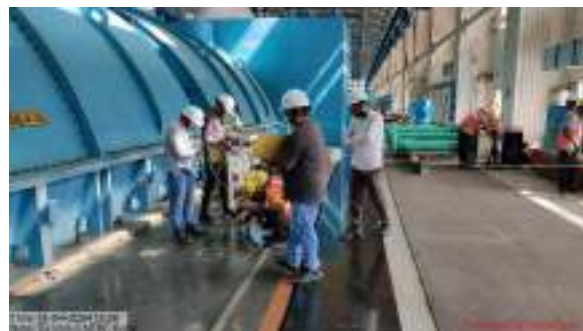
UPV Test on TG Deck Slab at NTPC Kudgi, Karnataka.
