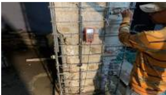
Continuity testing being done after installation of Zinc anodes at site of NHAI Residential Enclave at Dwarka, New Delhi
