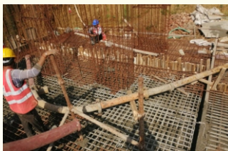
Central Public Works Dept. (Srinivaspuri, Delhi)
