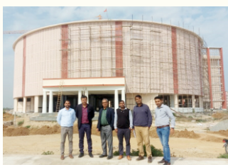
Construction of VC & Administration Building for Lala Lajpat Rai University for Veterinary and Animal Science at Hisar, Haryana
